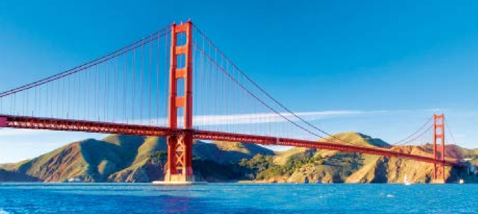
GOLDEN GATE BRIDGE
